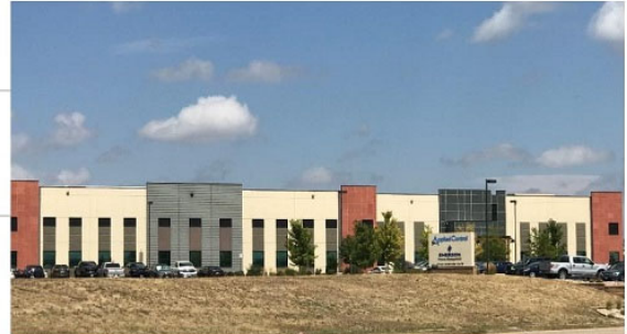
Applied Control Equipment – Denver, CO
